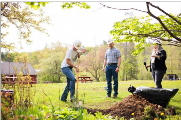
Rachel Stark breaks ground with a "golden" shovel, courtesy of the Spring Lake Ranch Shop Crew. Logistics Manager Nathan Hewitt buried a time capsule created by current Ranchers (shown wrapped in black plastic, bottom right) after Stark finished digging.
